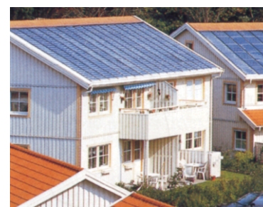
Figure 6.23: A solar panel fixed at the roof of a house.
