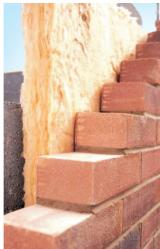
Figure 9.5: Soft insulation board between external brick wall of a Here A =  $20 \text{ m}^2$ house.
