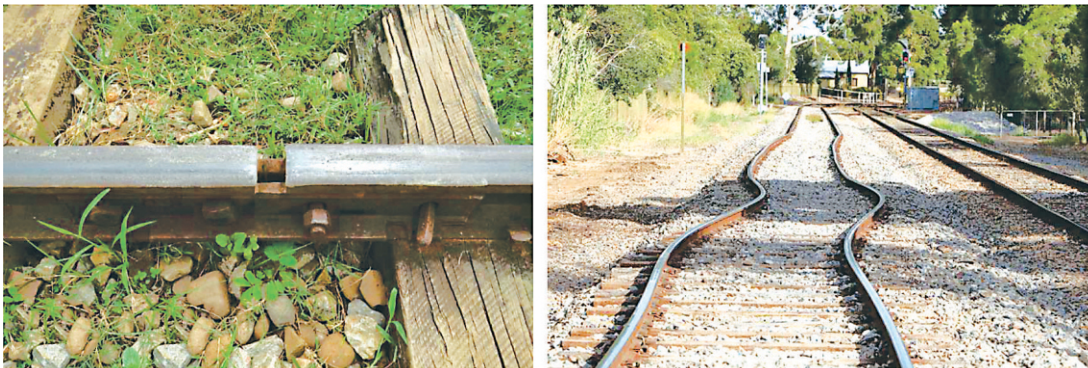
Expansion gap in railway track
