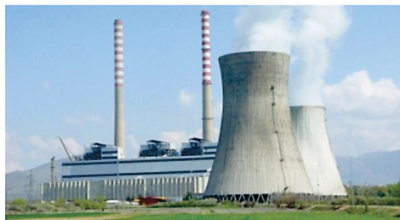
Figure 9.4: Thermal power plant
